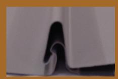
Snaplock panels fasten to the substrate through the manufactured pleated edge, which is then covered up by the next panel, which snaps in place as seen above. This allows for a hidden fastener appearance.
